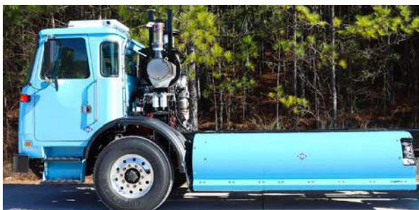
ACX FRAME RAIL INSTALL
