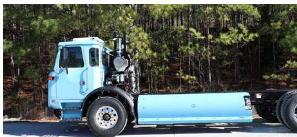
ACX FRAME RAIL INSTALL
